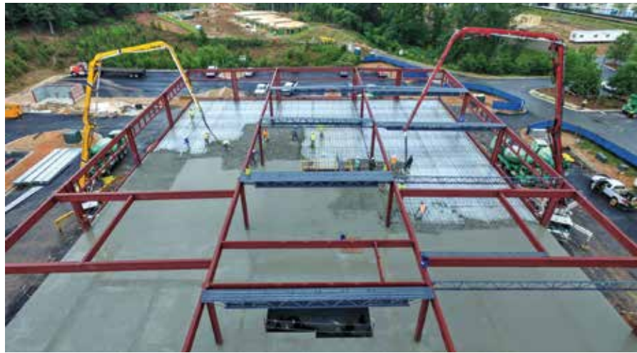
Pumping lightweight concrete onto a second story.
