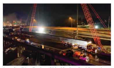
Cramped conditions dictating multiple pick points, plus girders maxing out just shy of 120 tons, prompted Guy F. Atkinson Construction to corral an unusually brawny crawler or telescoping crane fleet for erecting the final I-5 SB Puyallup River Bridge spans: 300-ton Manitowoc 2250, 650-ton Demag AT and 550-ton Grove. The contractor set a maximum 10 mph wind speed safety threshold for girder picks.
