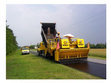
A chip seal crew working in Sampson County, applying STALITE lightweight road material over regular weight 78M. The road oil crews like the uniform application rates, on site delivery and reduced equipment stress that STALITE provides.
