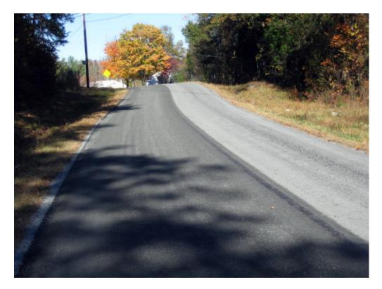
Shuping Mill Road in Rowan County, NC paved with Vulcan 78M on the right side with STALITE lightweight aggregate screenings applied as the second seal in the left side.
