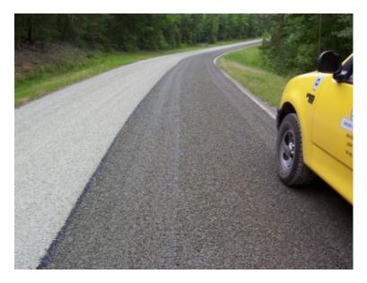
STALITE lightweight road material on the right lane and regular weight 78M on the left lane. STALITE is most often the material of choice in this area, since it can be applied as the ride surface without a blotting seal. This saves the cost of an extra step in the paving process. Also obvious is the darker color, which gives it an appearance much like plant mix asphalt.
